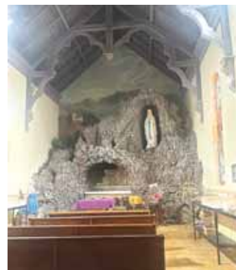
Grotto was built using bagasse clinkers (bricks) made from sugarcane. Bagasse is crushed sugarcane residue.
